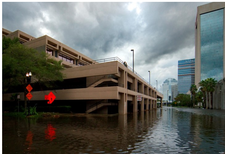
Figure 1. Hurricane Irma floods a parking garage and surrounding streets in Jacksonville, Florida. Infrastructure damaged during extreme weather events affects residents and businesses that rely either directly or indirectly on their services. Photo from iStock.
